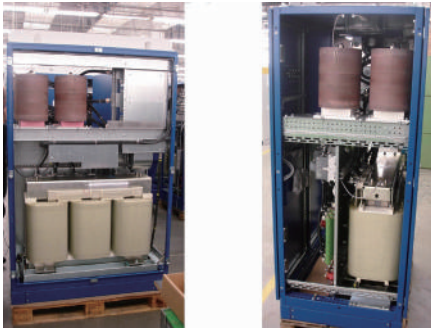
SGH Trafo in Zentralwechselrichter SGH transformer in central inverter
